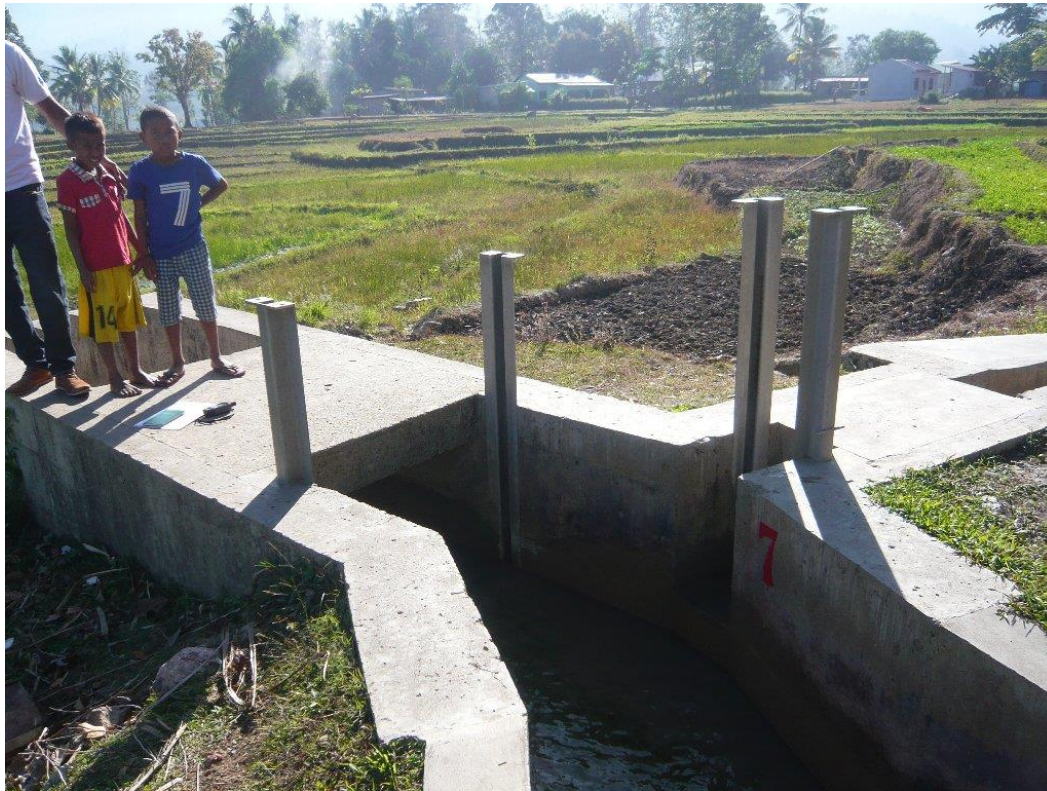
Both Sluice gates Removed (No.7, Ritabau)
