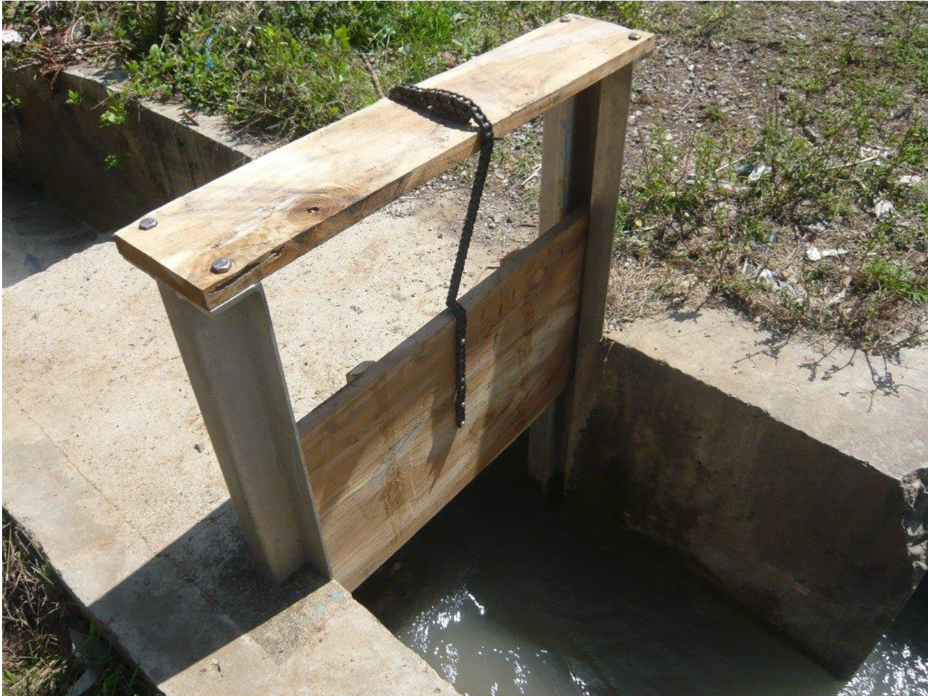
Wooden Stop log with chain
